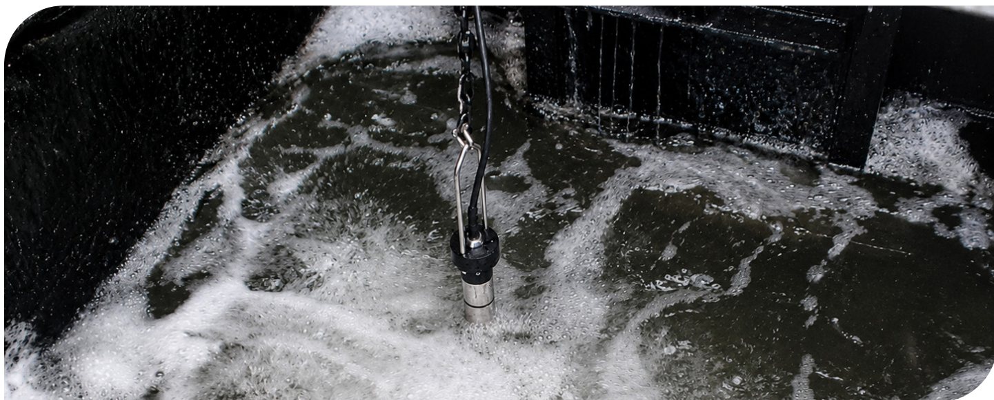
VARiON sensor deployed in the final effluent
